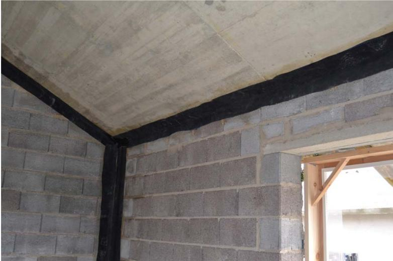
*Joints with rubber seal – source: M.Wassouf*
